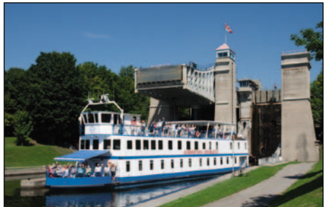
Peterborough Lift Lock
