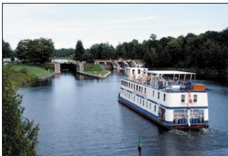
Talbot Lock and Dam
